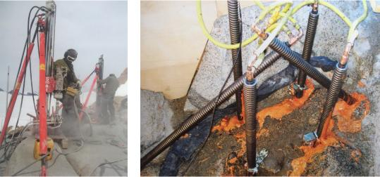
Figure 57. Drilling 6m deep holes in granite to install piles in preparation for steel pillars. Original author
