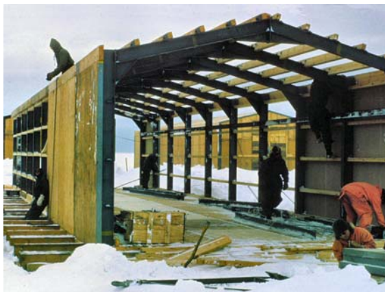
Picture above shows the timber grillage raft foundations and also the laminated timber beams, which weighed 16 cwt. each, to support the floor and steel portal frames. (E.J. Chinn)
