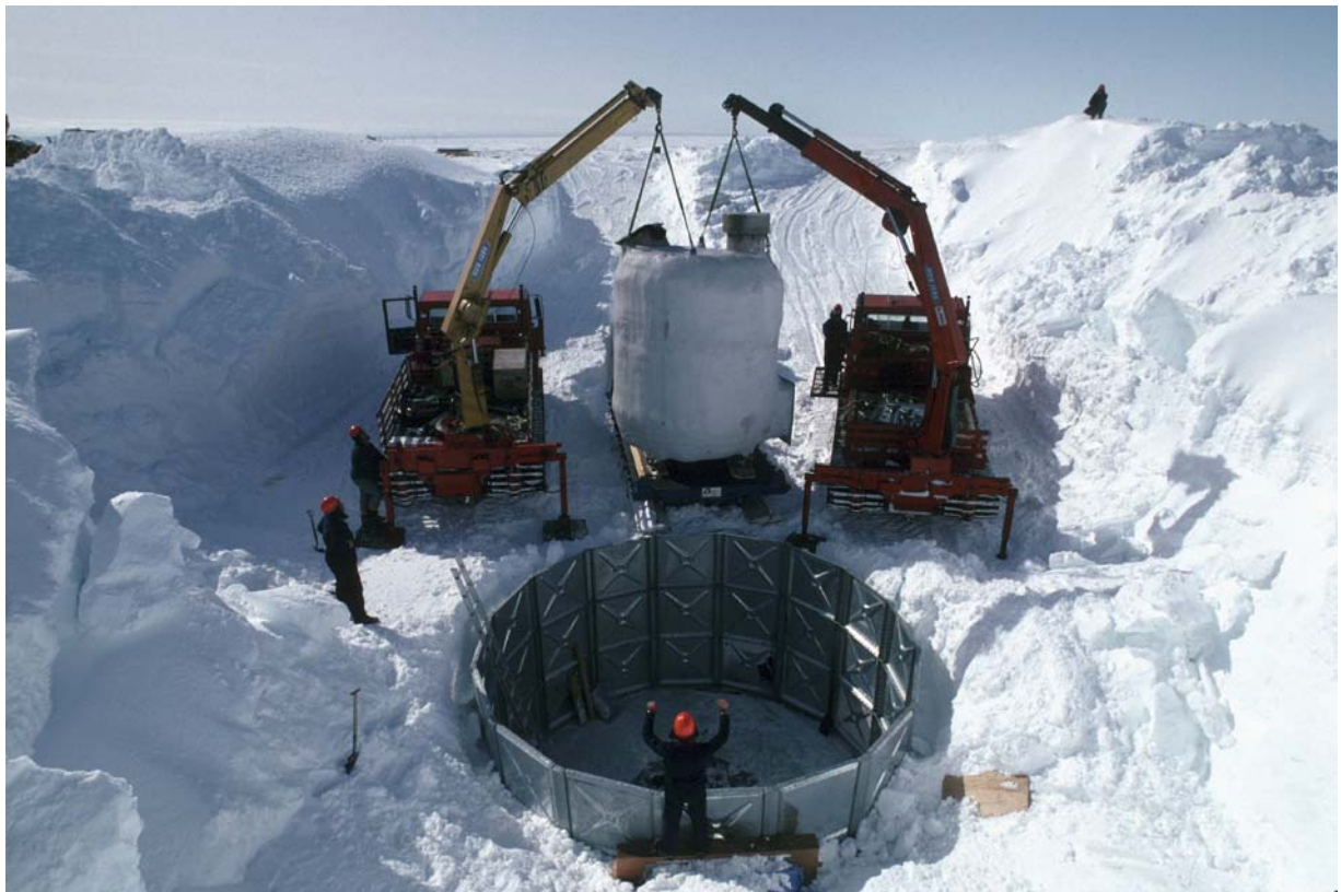
Above picture shows the replacement tank under construction 1992/93 season. (BAS)
