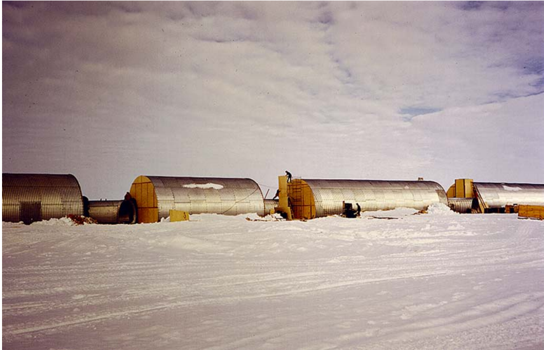
Armco completed (BAS)
