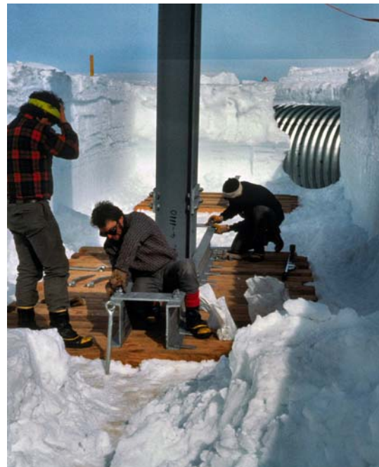
Timber and steel raft foundations (A Smith)
