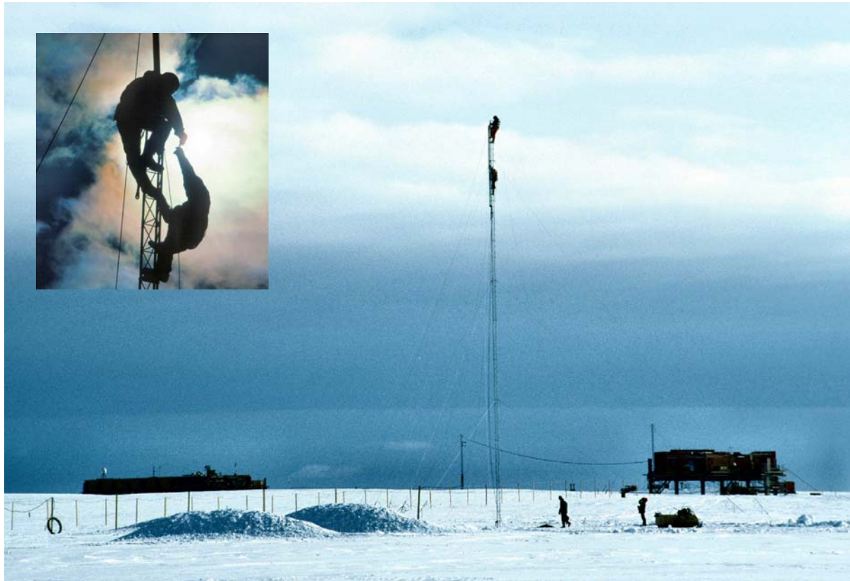
Above picture shows the erection of a scientific mast (BAS)
