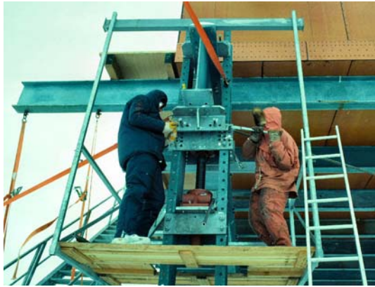
Picture to the left shows the jacking operations February 1990 (A. Smith)
