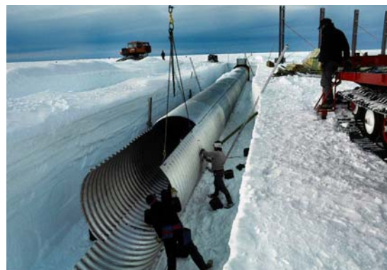
Armco tunnel connecting ACB to ICB (A. Smith)
