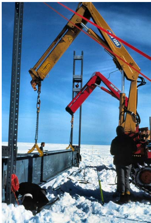
Picture to the right shows platform manual jacking system. This system was changed to a mechanical system at a later date. (A. Smith)
