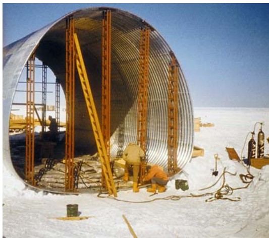
Picture to the left shows the gable end in course of erection.
