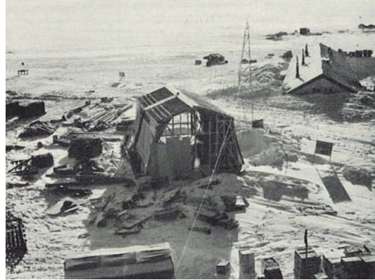
Partially constructed generator shed from the north-west in 1957.
