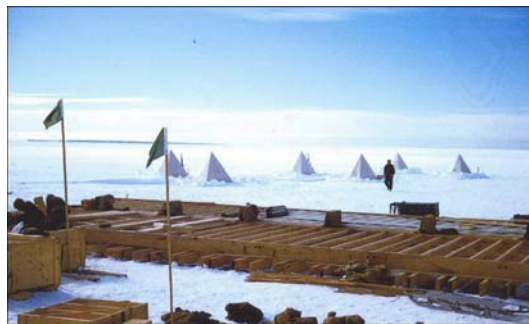
Main hut foundations (D.W.S. Limbert)
