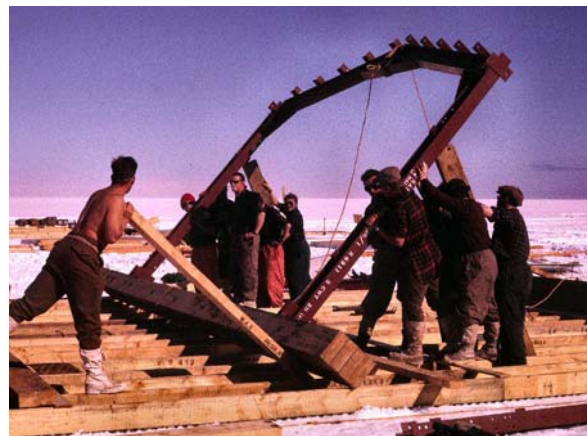
Picture above shows the timber grillage raft foundations and also the laminated timber beams, which weighed 16 cwt. each, to support the floor and steel portal frames. (E.J. Chinn)
